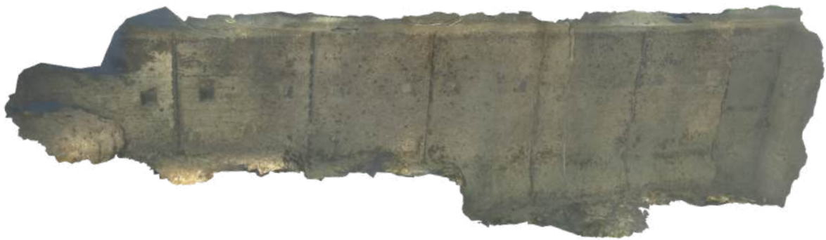
3D model - Quay wall inspected with Hydro 100
